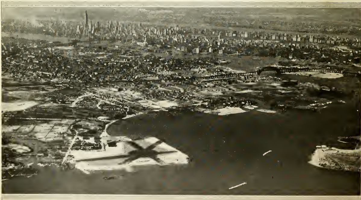
Near the shadows of Manhattan's tall towers, Glenn Curtiss Airport is a fitting reminder of an illustrious pioneer
